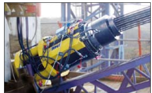
▼ Two concrete arches of this viaduct in Silleda, Spain are rotated and lowered by Enerpac Heavy Lifting Strand Jacking Systems.
