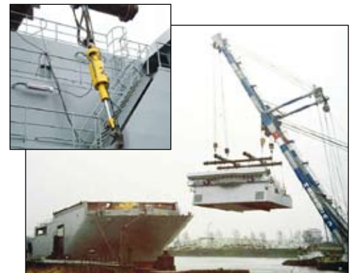
▲ Perfectly synchronised balance: Naval ship superstructure weighing over 600 tons placed on the hull using Enerpac's hydraulic SyncHoist.
